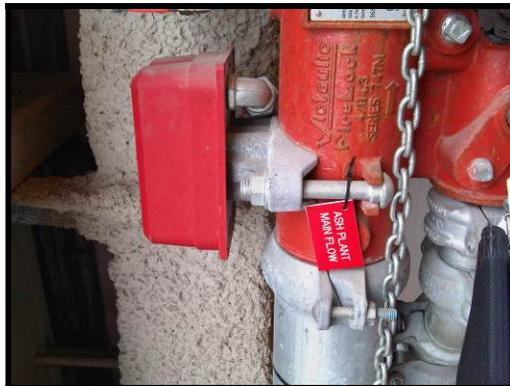
**Image 24: Sprinkler System Flow Switch**
