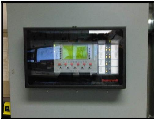
**Image 21: Main Fire Alarm Control Panel**
