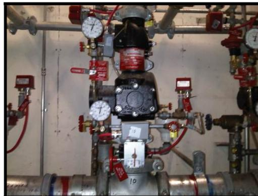
**Image 2: Preaction Sprinkler System Riser**
