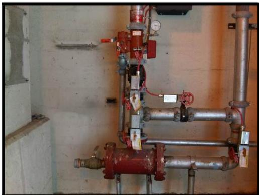
**Image 1: Wet Pipe Sprinkler System Riser**
